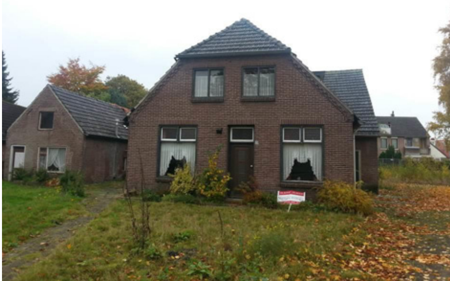
Foto 1: te slopen woning.
