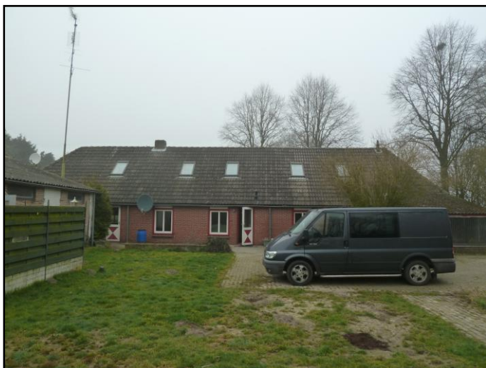
Te slopen woning
